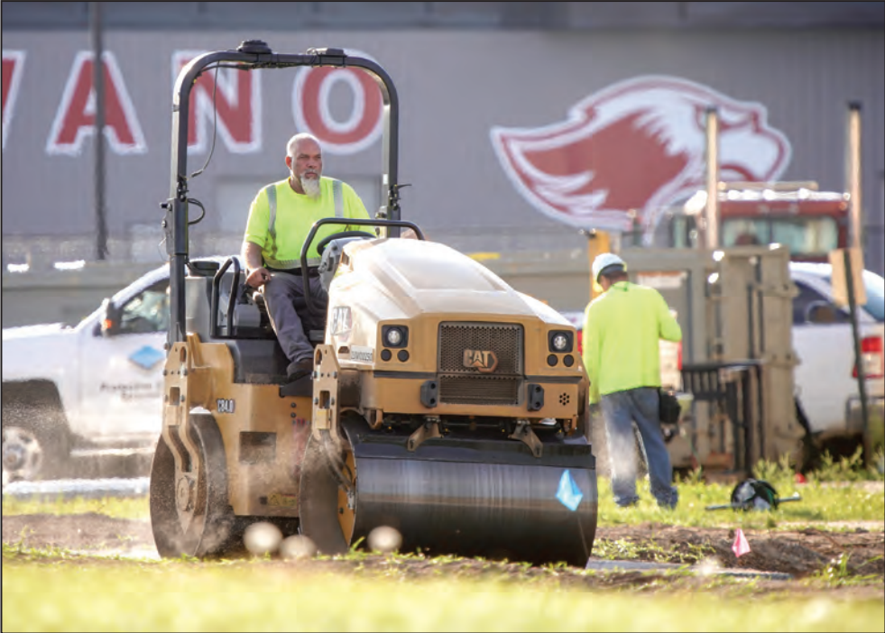
Construction crews were out in full force preparing the Shawano Community High School sports stadium, parking lots and driveways in advance of the first soccer and football games. While the soccer team lost 2-0 to Ashwaubenon on Aug. 25, the football team beat Lakeland Union 16-15 on Aug. 28.
