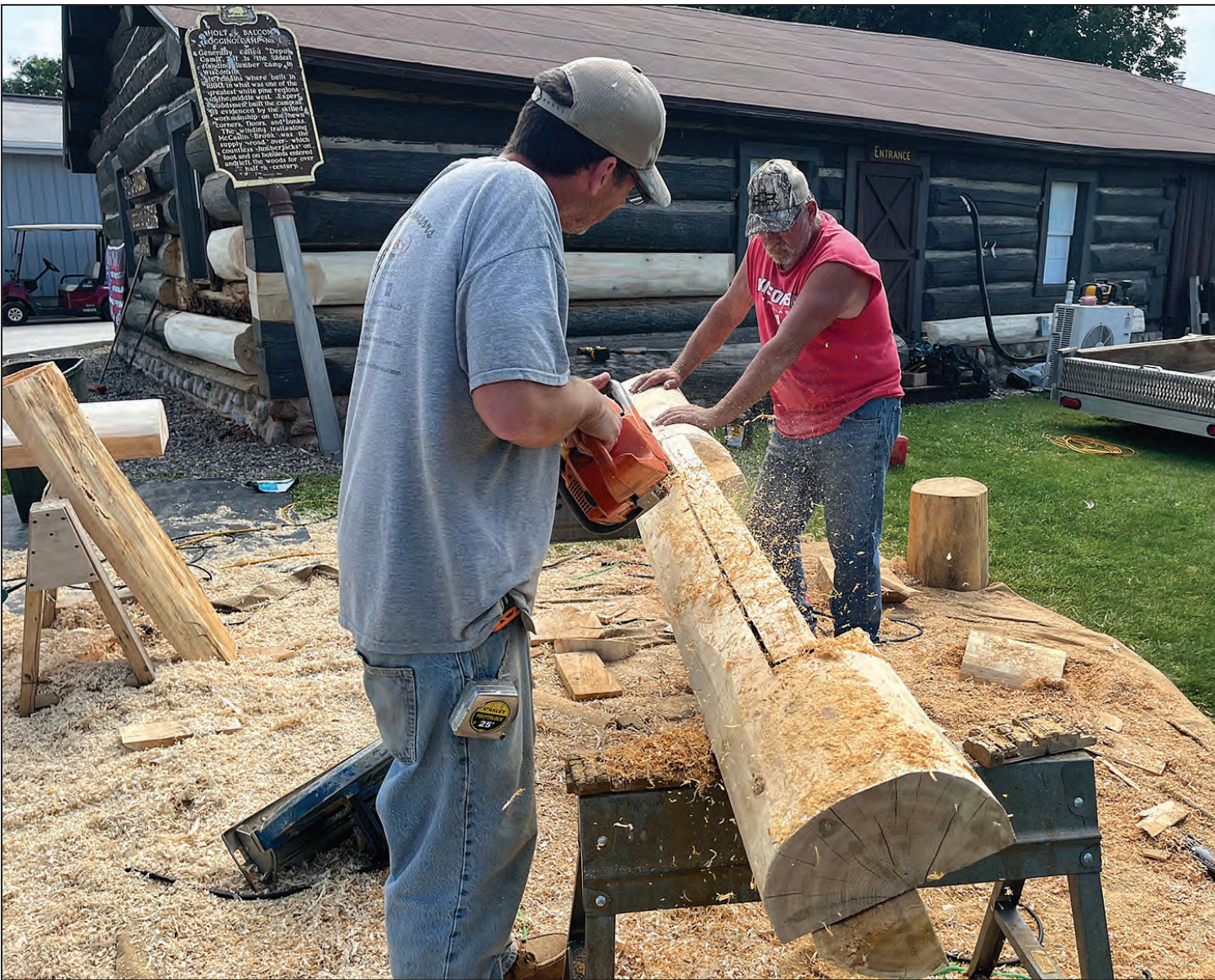
BALCOM, continued on page 2 Mountain Log Homes technicians did extensive repairs to the Holt and Balcom Logging Camp in August. JON MARSH
