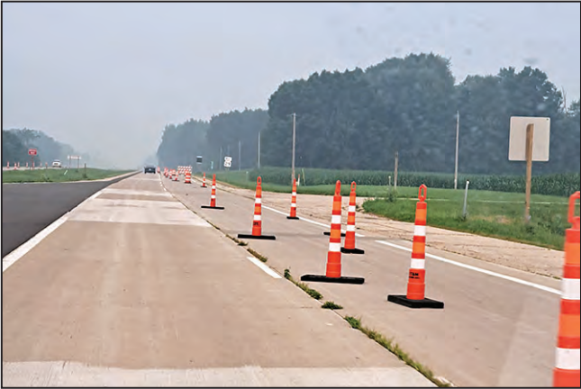
Eastbound and westbound traffic on state Highway 29 is limited to one lane for much of Shawano County, as the Wisconsin Department of Transportation works on several reconstruction projects.
