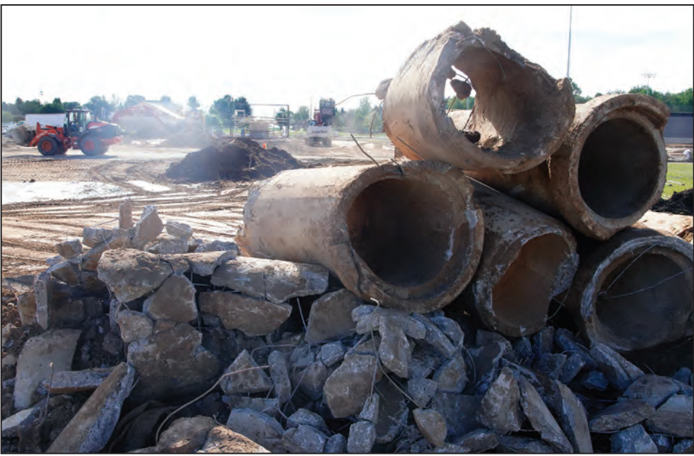
An average of 120 workers are on site every day at Shawano Community High School. Crews are touching nearly every square foot of the building as well work in the parking lot and athletic complex.
