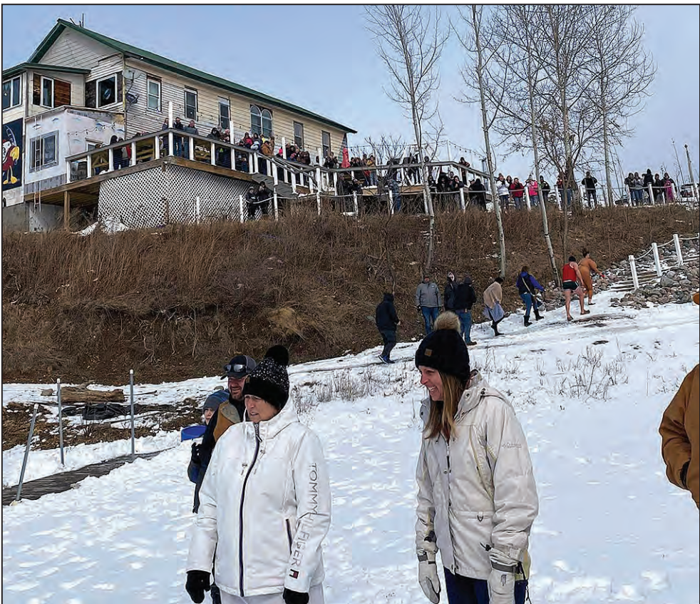
Little Topsy is the oldest commercial building in Townsend and one of the funner places in the town, but a catastrophic water leak has closed the original Wheeler Hotel while repairs are made, impacting the building's summer revenue potential.
