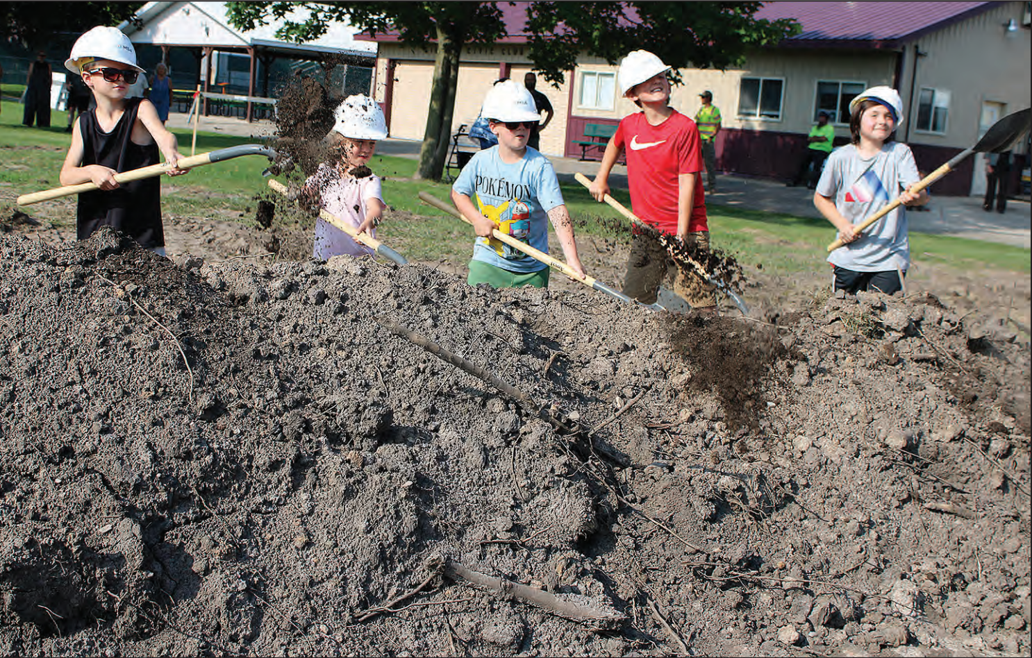
Some of the children of Gillett toss dirt during the July 8 groundbreaking ceremony at Zippel Park. The new playground is expected to be finished in October and will replace the old playground, which has some equipment that's 70 years old.
