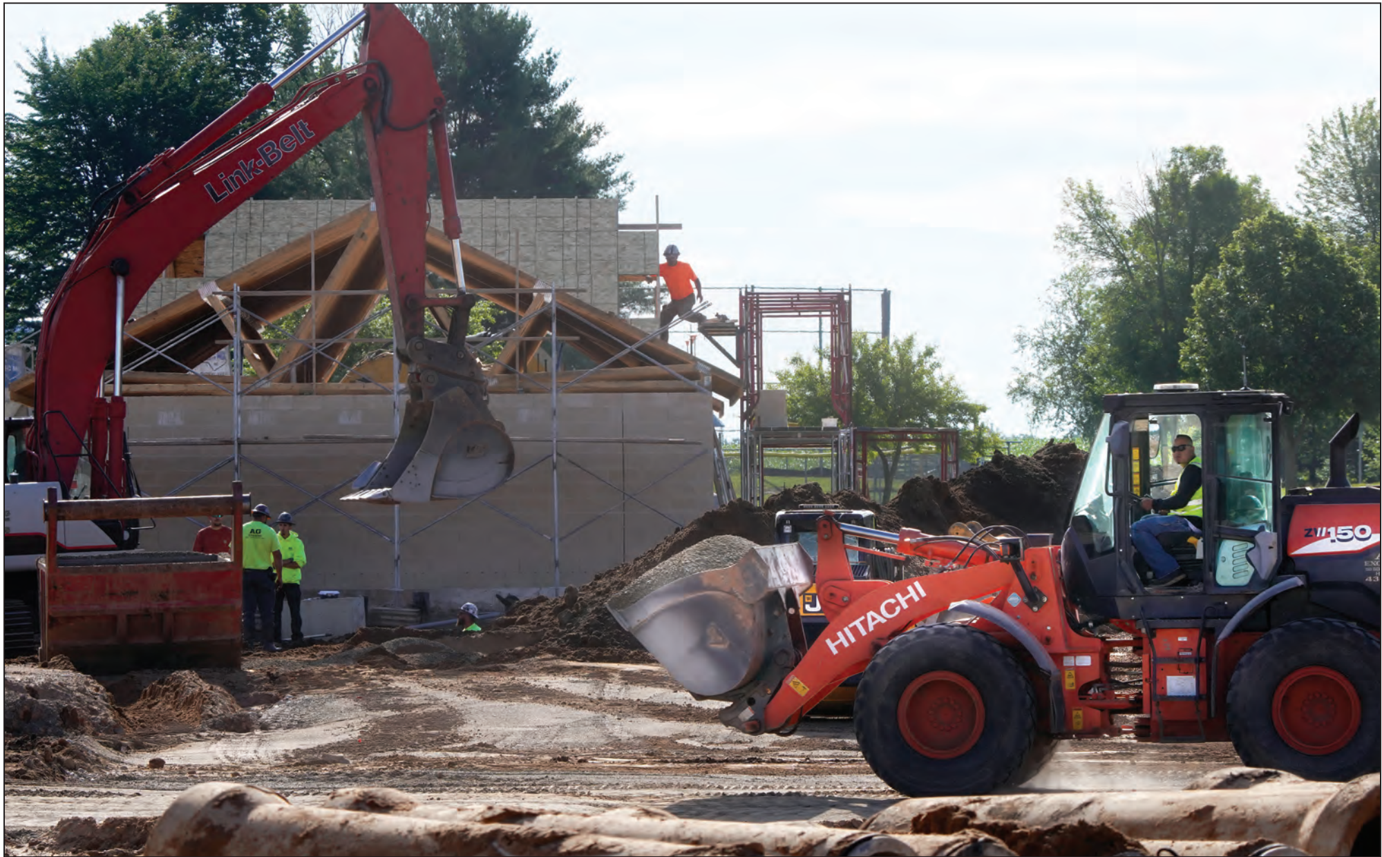
Crews are busy at it this summer at Shawano Community High School, preparing the school and the athletic facilities for the fall of 2026. The football field is nearly ready, with the track around it, bleachers, storage and press box in place. Construction continues on the concession stand and ticket booth.
