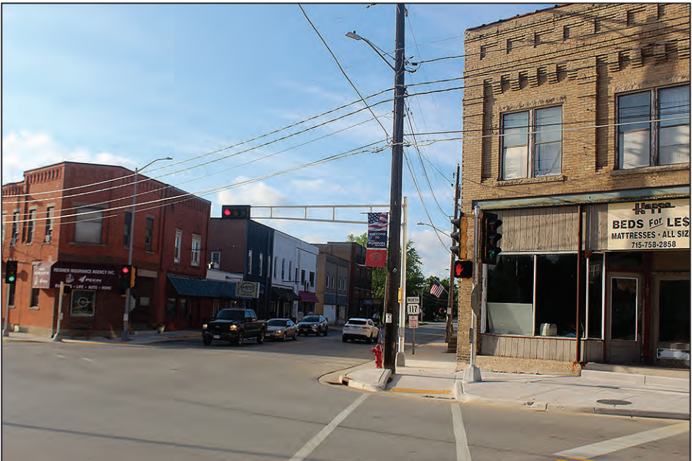
Closed buildings, like the one on the right on Green Bay Street in Bonduel, are ones that the Bonduel Redevelopment Authority seeks to revive. Ideas were tossed about June 9 on what the authority could do to make its downtown thrive again.
