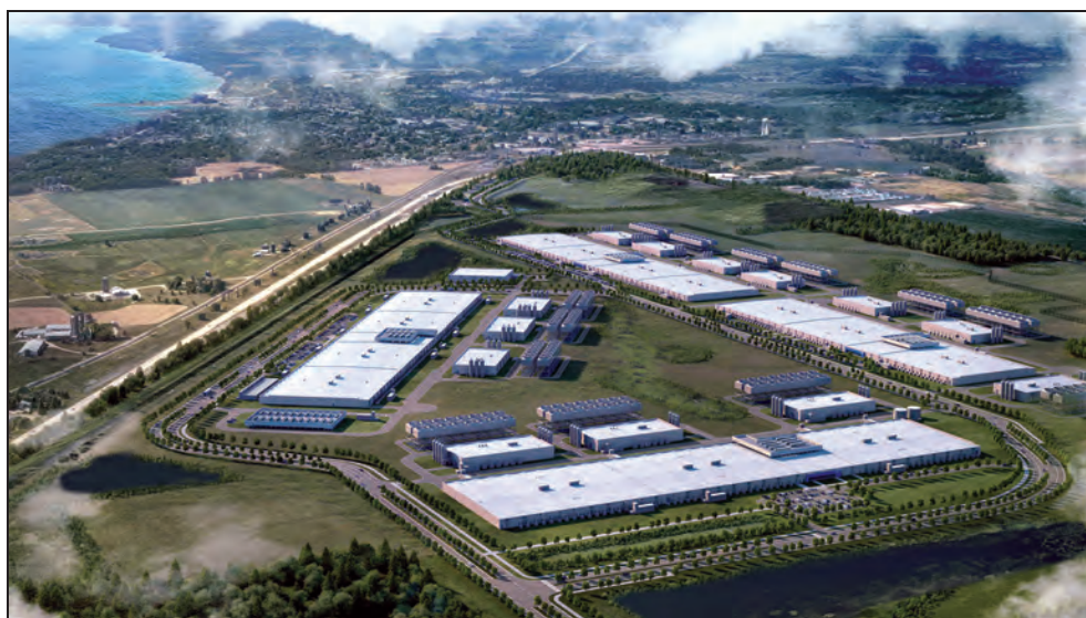
This is a rendering with a southwest view of the Lighthouse campus, a massive $15 billion-plus artificial intelligence data center located in Port Washington. Developed by Vantage Data Centers with major tech tenants OpenAI and Oracle, the 672-acre campus is scheduled for completion in 2028.
