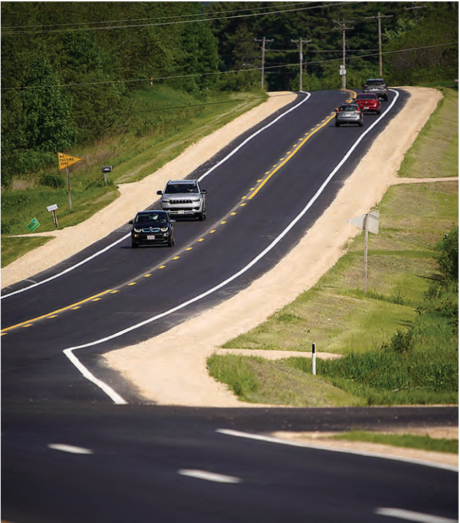
County Road BE between Shawano and Bonduel is open to traffic once again following the successful repaving of the roadway. Many drivers use it as a way to avoid the reconstruction work going on along state Highway 29 between the two communities. GREG MELLIS | NEW MEDIA
