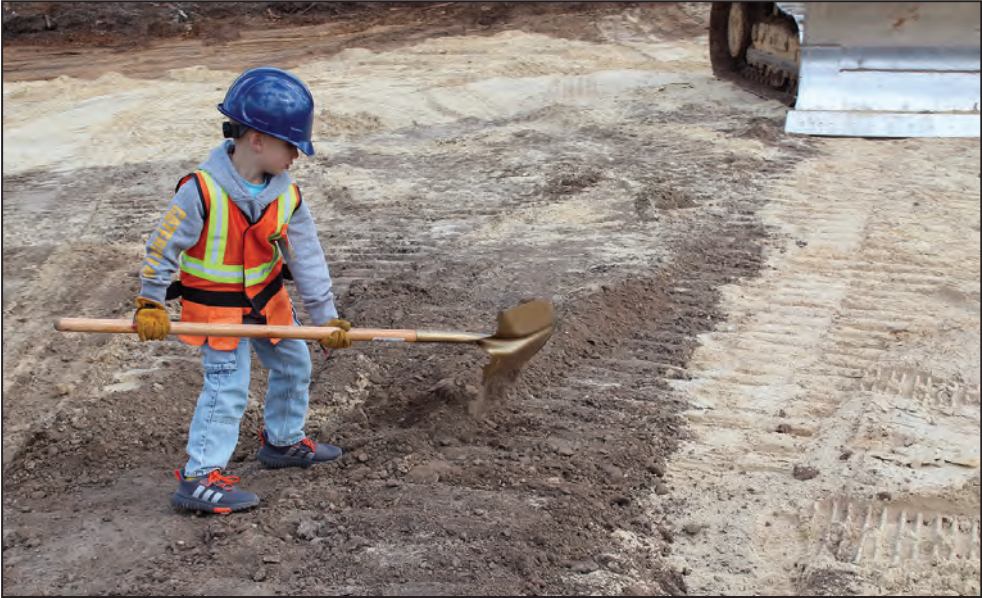
Caden Stevens, son of Andrew and Dr. Rebecca Stevens, didn’t wait for the May 6 ground-breaking ceremony to begin before starting to dig into the dirt for the new dental office at 3000 S. Airport Road.
