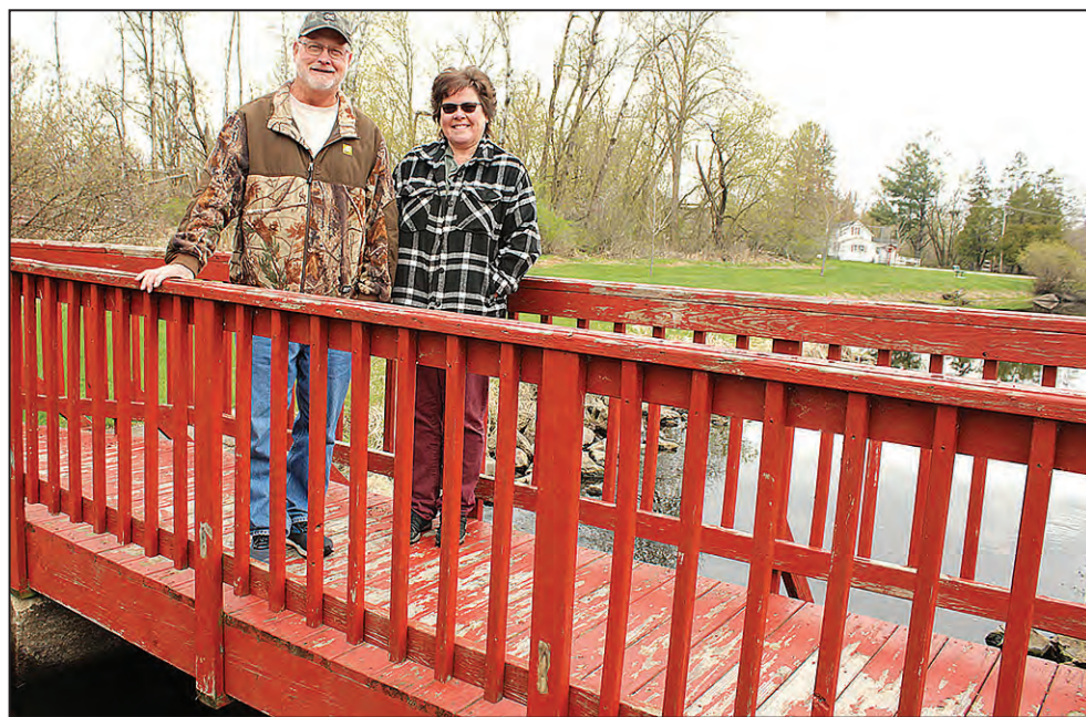
Eland Village Board Trustee Howard Graves and Village Clerk Denise Larson stand on a bridge that's part of a dam that forms Eland Mill Pond. The dam is in need of repairs and the village recently started a fundraising effort for the project.
