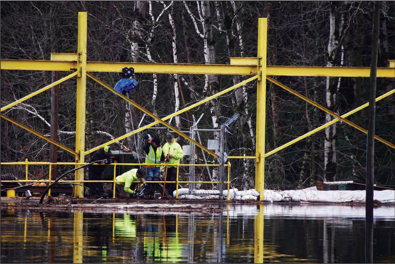
With sandbags piled on the sides of the Balsam Row Road Dam, workers clear debris that is blocking water from flowing through the dam in mid-April. County highway workers built sand berms on each side of the dam to force the water over the dam rather than flooding onto the embankments on each side.
