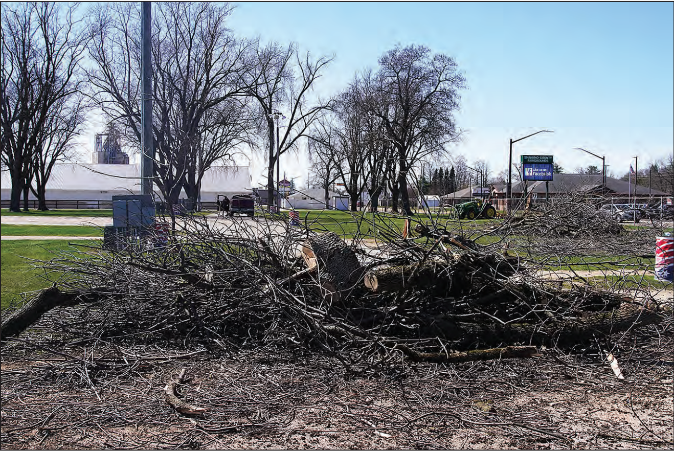
Kopitzke Logging, of Tigerton, removed 27 ash trees from the Shawano County Fairgrounds the week of April 20. The work also included grinding down the stumps and removing all of the debris. Trees may be replanted after the 2026 Shawano County Fair, and officials will investigate whether any grant money is available to help cover that cost.
