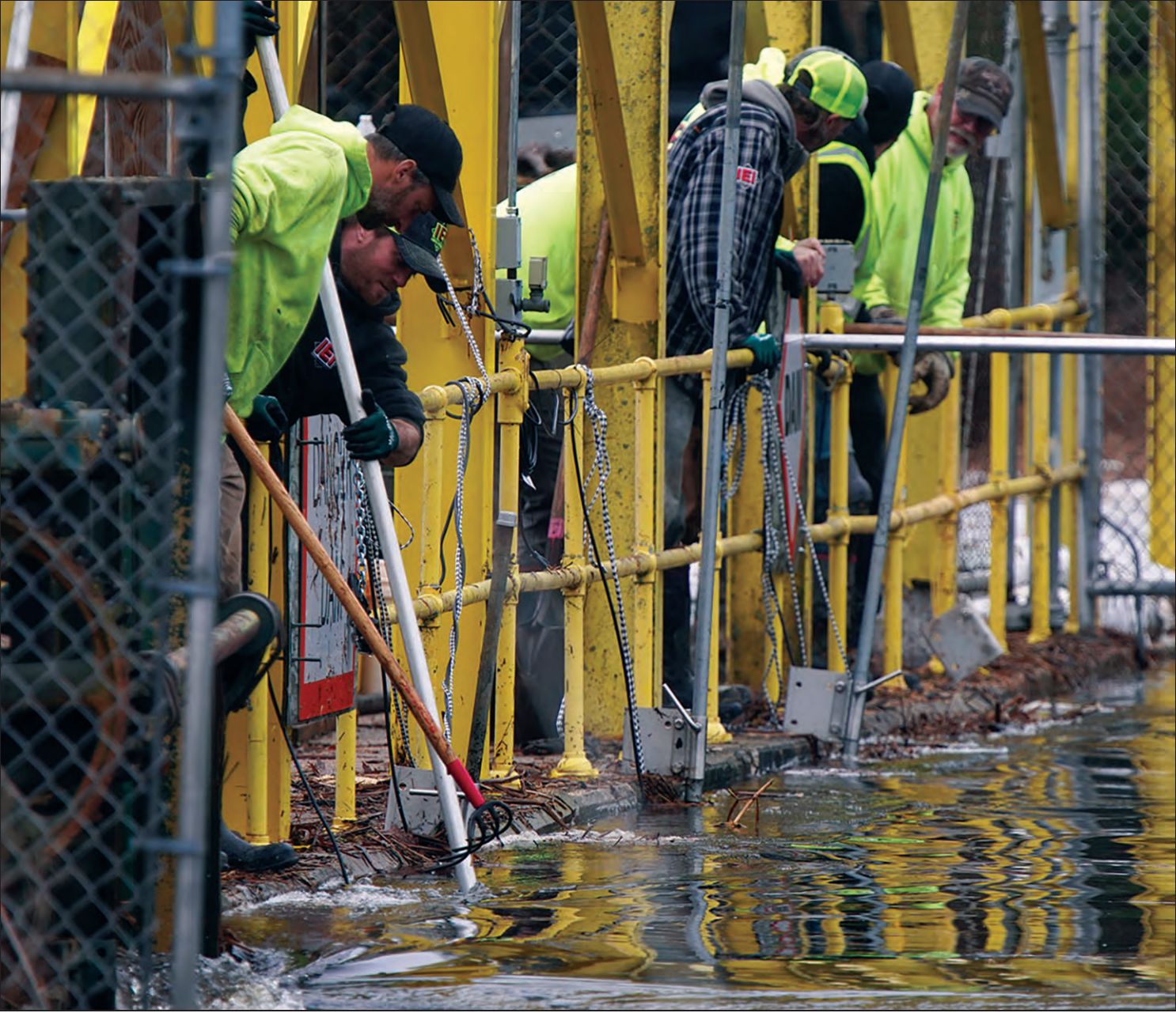
Crews work to remove large branches and other objects from blocking the flow of water at the Balsam Row Road Dam on April 15. Shawano County Highway Department workers installed sand berms on each side of the dam to force any flood water to go over the concrete dam and not alongside it onto the shore.
