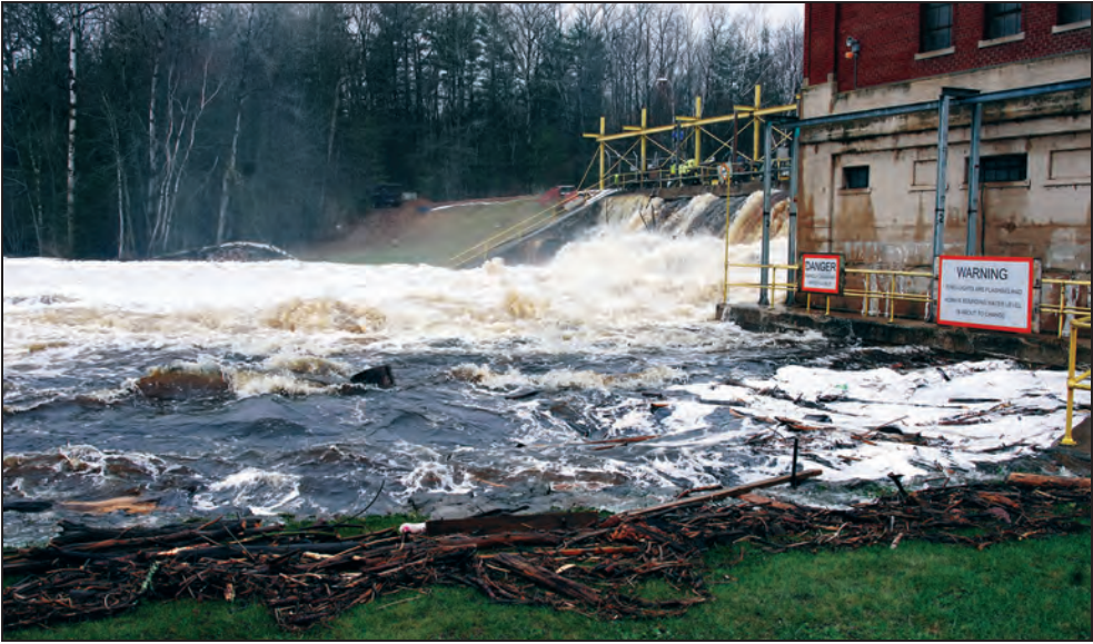
Communities in Shawano, Menominee, Oconto and Outagamie counties and more continue to be on watch due to historic flooding that has led to evacuations, closures and infrastructure breakdowns.
