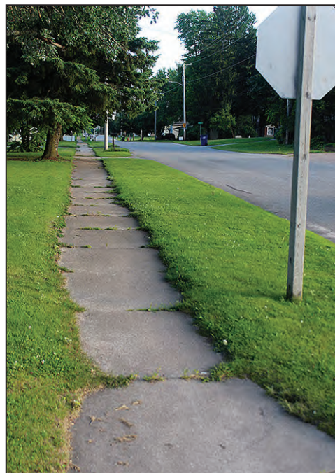
A portion of South Ellms Street will receive new sidewalk this year, although that segment is later in the schedule.
