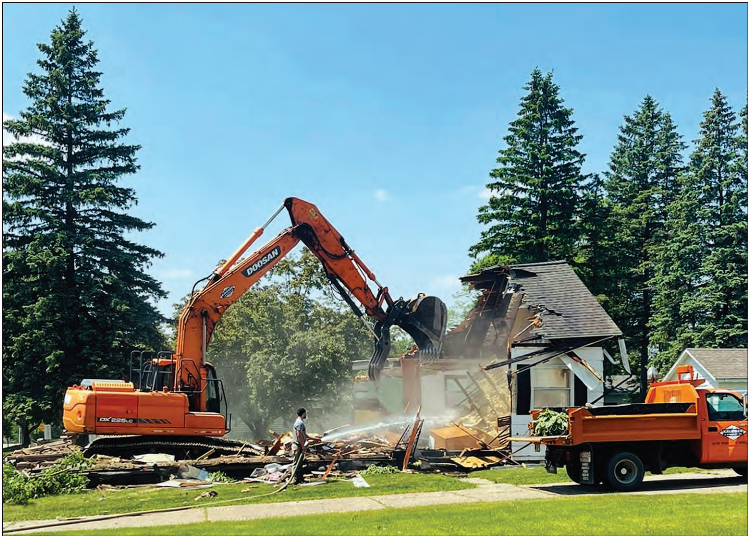
Calvary Lutheran Church in Antigo purchased the adjoining property from Peace Lutheran a year ago. The home, in need of expensive renovation, was razed June 4, anticipating the expansion of the fellowship hall and renovation of the kitchen.
