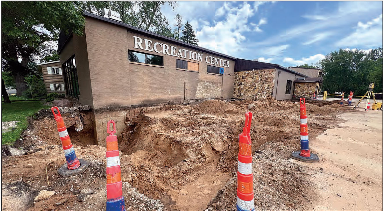
The reconstruction of the Shawano Recreation Center is underway, inside and outside. The center is expected to reopen in the late spring of 2026. GREG MELLIS | NEW MEDIA
