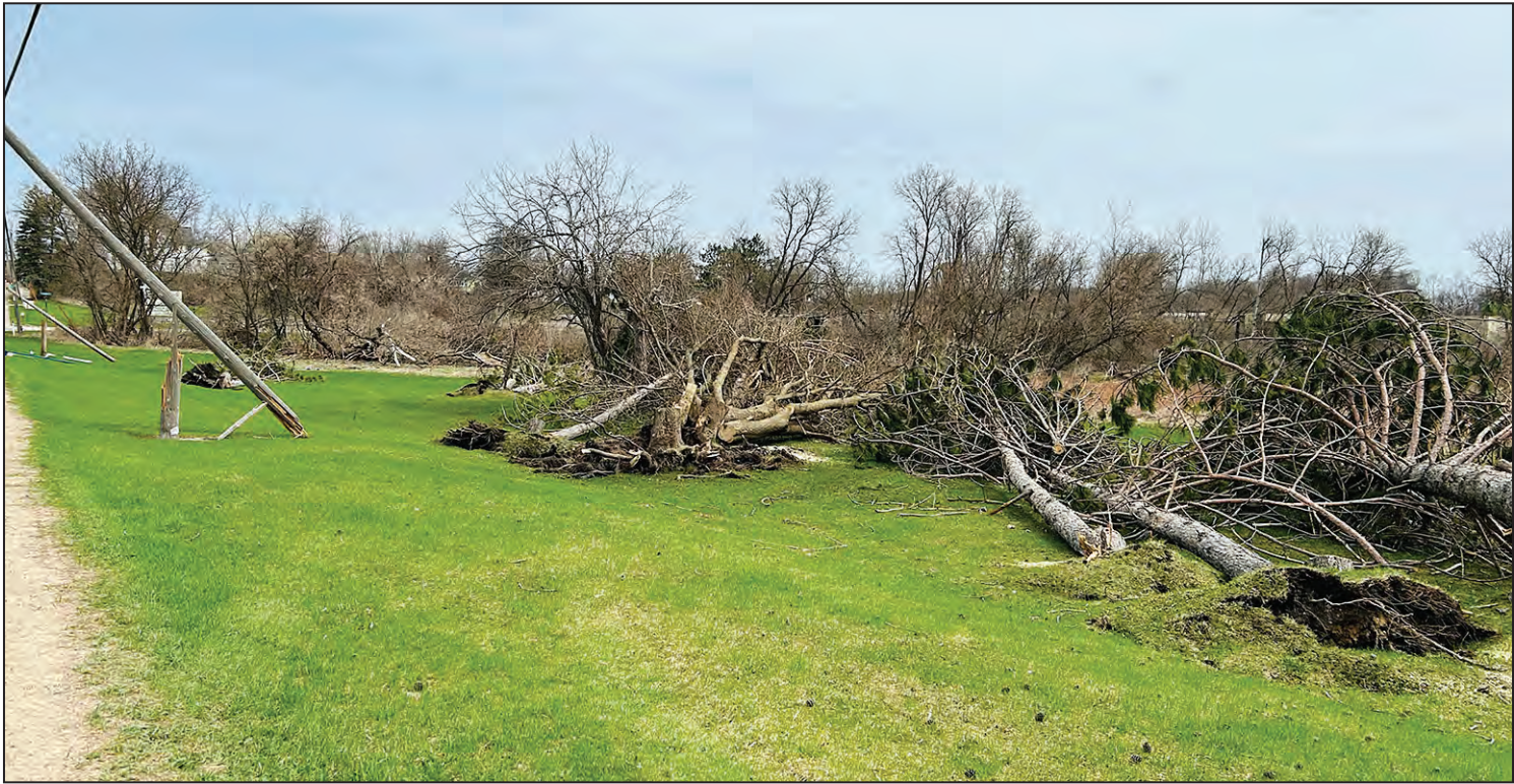
Power poles and trees were flattened on the south end of Mattoon as winds reached 80 mph the night of April 28. Crews were out the next day repairing the damage. LAUREL COLLINS
