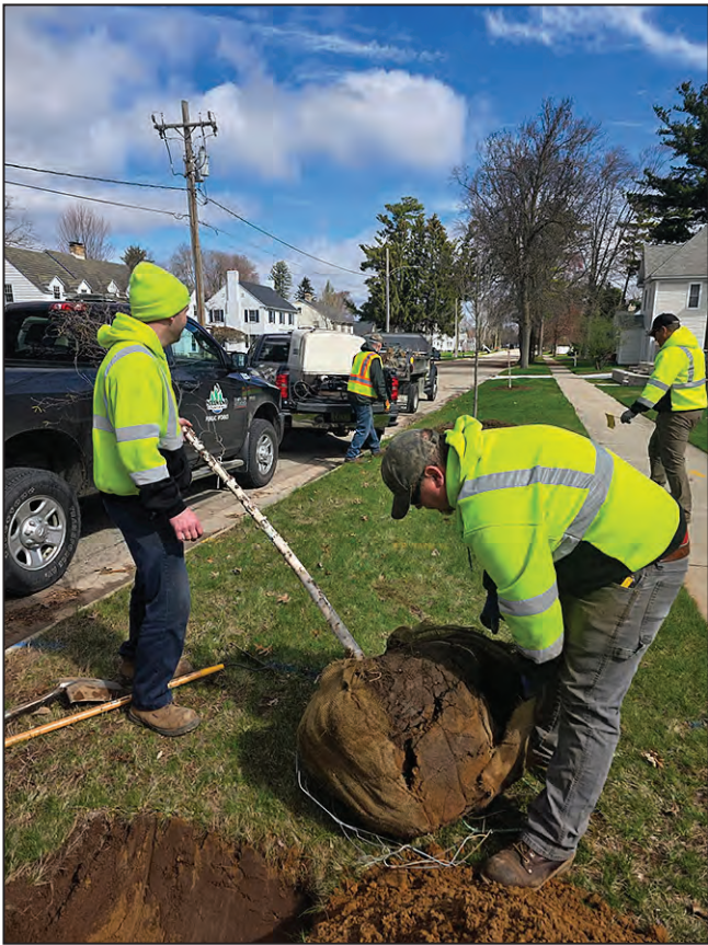
City crews put in an elm tree on South Bartlett Street, one of dozens of trees it plants annually in Shawano.
