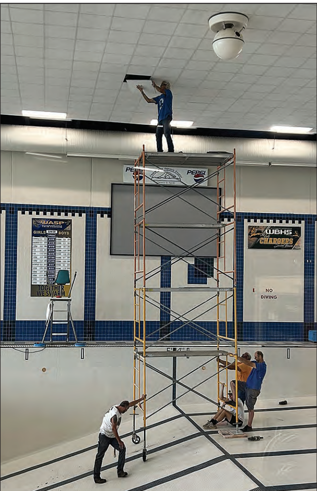
Steve Vera replaces tiles at the Darwin E. Smith Aquatic Center during its recent renovation. The pool is celebrating its 25-year anniversary.
