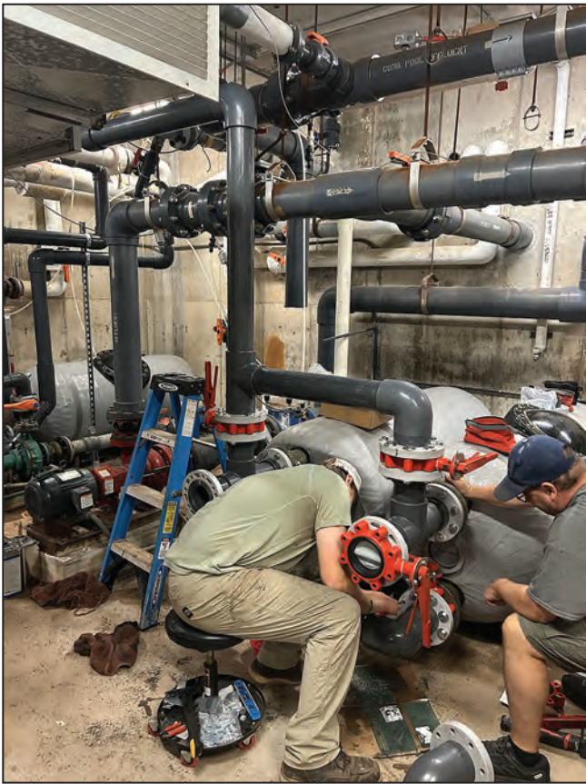
Workers replace equipment during the recent renovation and repair project at the Wittenberg-Birnamwood High School pool. Repairs and maintenance projects were made possible by using investment earnings from the Darwin E. Smith Community Aquatic Center Endowment Fund, totaling $250,000. CONTRIBUTED
