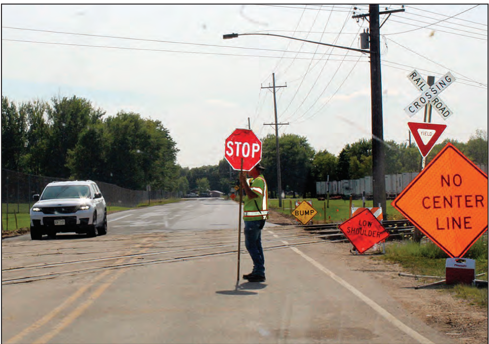
An SUV exits the newly blacktopped portion of County Road MM west of Shawano on Aug. 14. Shawano County Highway Department crews performed the work on the 0.25-miles section of road, along with several other similar projects. KEVIN PASSON | NEW MEDIA
