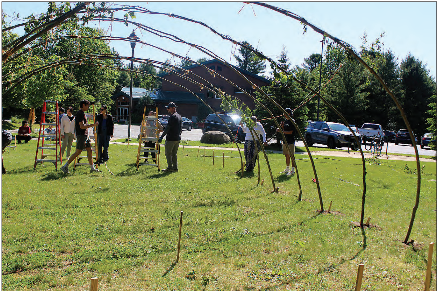
Work from the first day on the new teaching lodge frames the interns and community members as they embark on the second day of construction May 30 at the College of Menominee Nation's Keshena campus.
