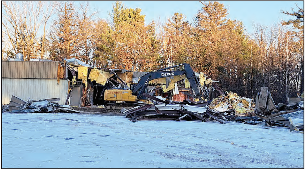
Demolition crews are razing the former The Gathering banquet hall and restaurant at 2600 E. Richmond St. In 2024, it was purchased by Charter Aarrowcast, which is directly east of the restaurant. Charter Aarrowcast produces ductile and gray iron castings for customers in various industries. From government and defense customers to agricultural and heavy truck equipment manufacturers, and an array of companies that need pumps, valves and compressors, Charter Aarrowcast creates custom castings.
