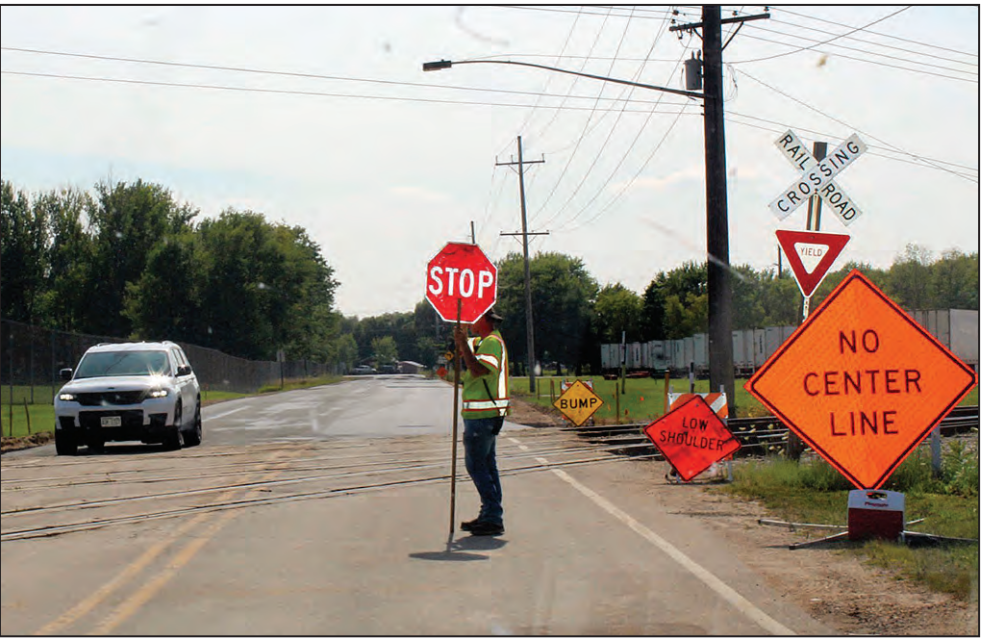
An SUV exits the newly blacktopped portion of County Road MM west of Shawano on Aug. 14. Shawano County Highway Department crews performed the work on the 0.25-miles section of road, along with several other similar projects.
