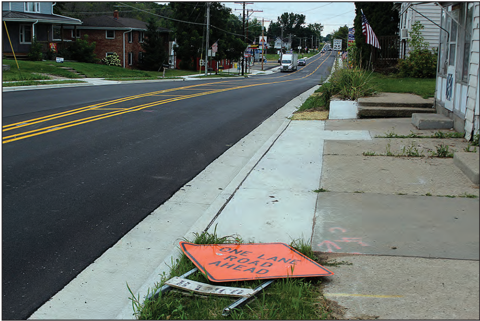
A sign warning about a one-lane road ahead lies on the sidewalk, no longer needed Aug. 8 as traffic returns to normal on state Highway 117 in Bonduel.
