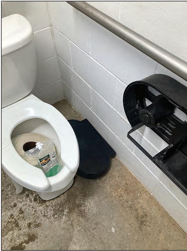
A roll of toilet paper and a package of soap were stuffed into a toilet recently at the restrooms by Naberhood Plaza and Franklin Park. The Shawano Police Department is seeing an increase in park vandalism, as well as a number of other juvenile crimes. CONTRIBUTED
