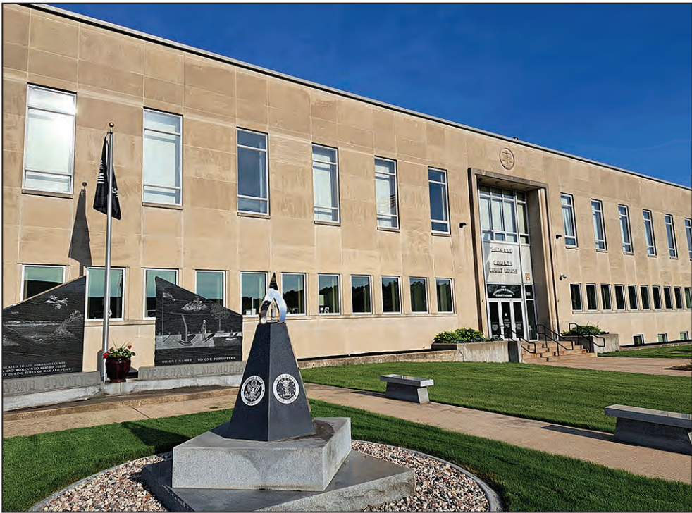
The Shawano County Courthouse was built nearly 70 years ago and is in need of millions of dollars of repairs and improvements, according to county officials. County supervisors will soon consider whether to create a master plan for all county properties.
