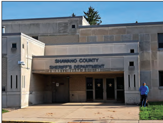
The Shawano County Sheriff's Department and Jail were the subject of a recent facilities assessment that indicated significant repairs and improvements are needed. Also, inmates are routinely walked across the street and through the hallways of the courthouse when they need to appear in court, creating a safety issue for the inmates, staff and the public.
