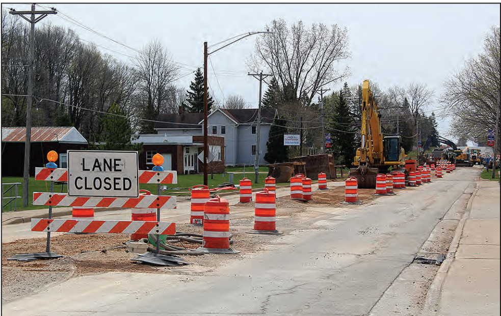
The state Highway 117 reconstruction work has reached into Bonduel’s business district, with through travel prohibited but allowing for access to businesses along the way. The normally busy highway has seen traffic drop down to a trickle, according to Jesse Rankin, the village’s municipal operations director. LEE PULASKI | NEW MEDIA
