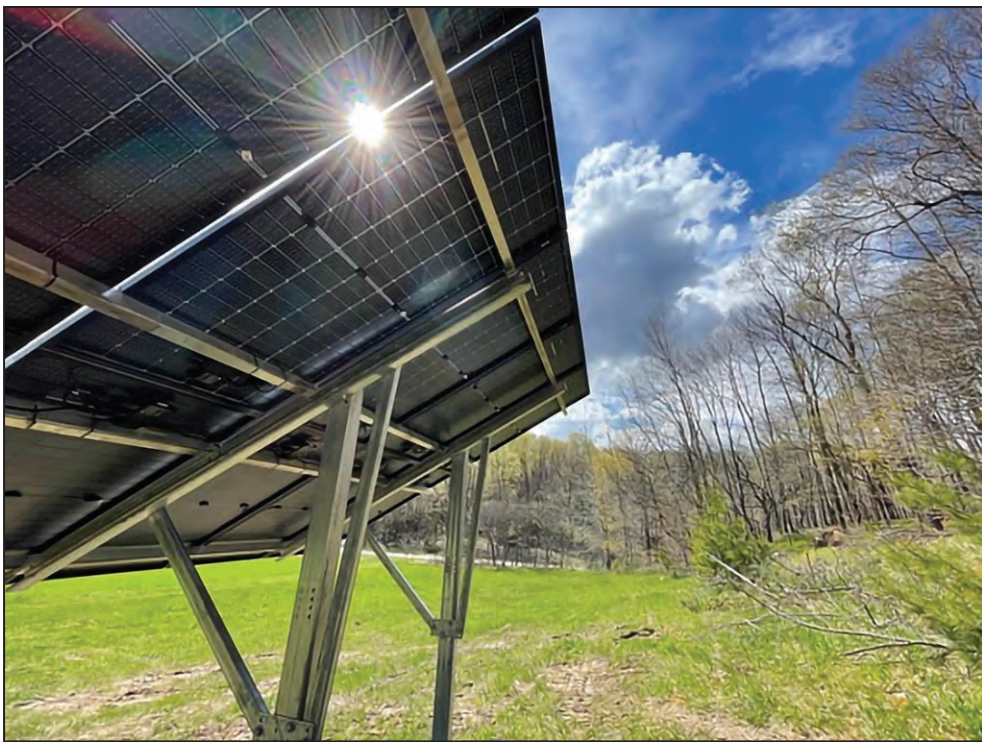
A newly installed solar array stands in a field in Marion. This small array will save a local cabinet manufacturer $981 per year, replacing 89% of the company's energy use. TEGAN GRIFFITH
