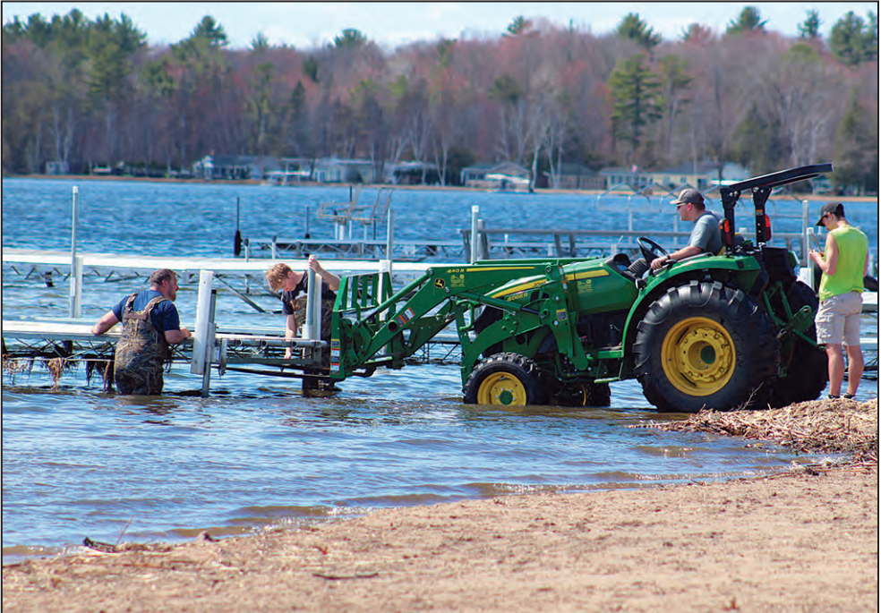
Warm temperatures on April 14 didn't go to waste as crews spent part of the day installing docks at Shawano Lake County Park. Dozens of others showed up to have picnics, bask in the sun, jump in the water and play with their dogs.
