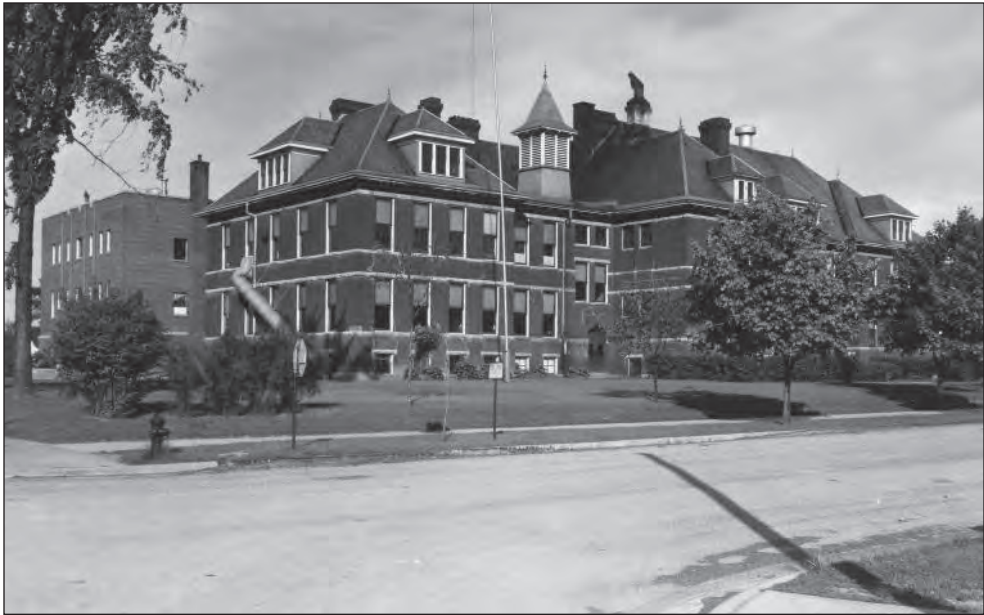
A view of the Oconto Falls High School building that was constructed in 1902 along with classroom additions from 1914 and, in the background, the Central Avenue gymnasium, which also housed classrooms on the first floor underneath the second-floor gym. The gymnasium survived a 1957 fire that gutted the original school buildings.
