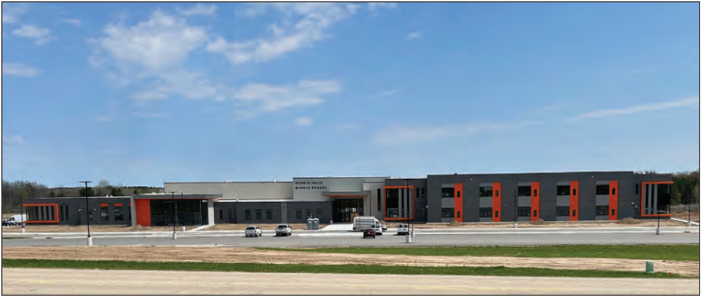
District officials say construction of the new Oconto Falls Middle School is ahead of schedule and under budget. WARREN BLUHM | NEW MEDIA
