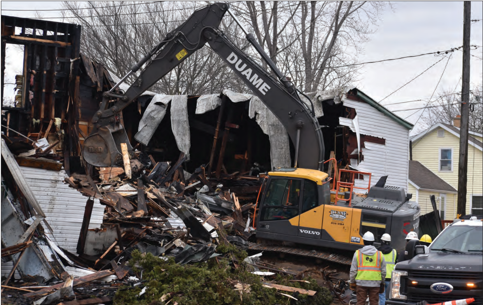
An excavator from Duame Sand and Gravel removes debris under the direction of Oconto fire investigators Feb. 27, the morning after a blaze that gutted the two-story structure at 1131 Main St. WARREN BLUHM | NEW MEDIA
