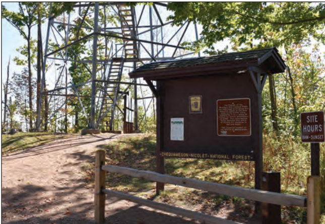
Workers cleared brush to better define the parking lot and erected a split-rail fence to protect the information board at the Mountain Fire Lookout Tower this summer.
