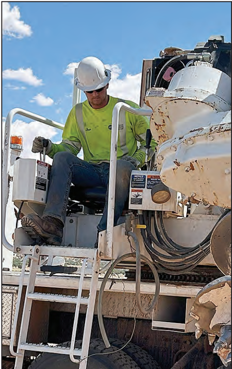
Central Wisconsin Electric Cooperative lineman Josh Wick operates a pressure digger. Most of the pole holes required a pressure digger because of rock in the area.
