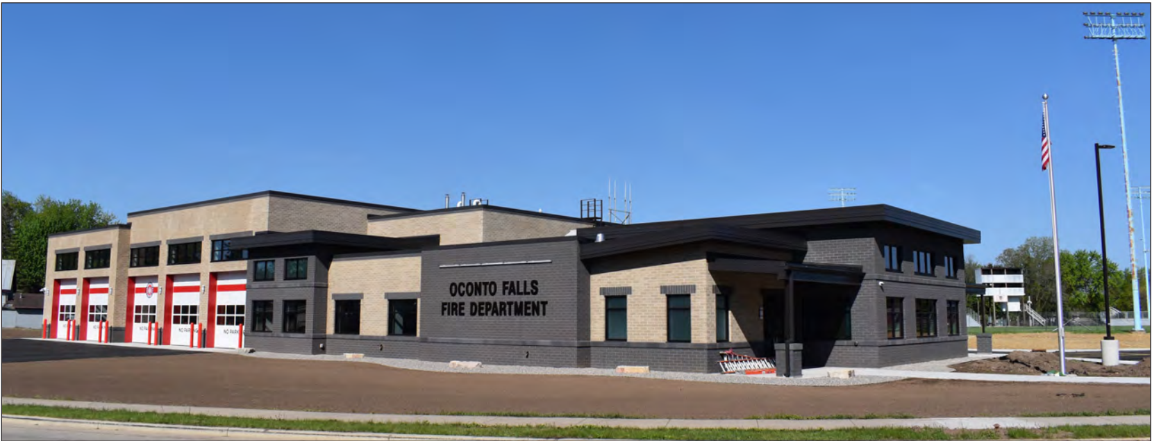
Contractors were scheduled to release the new Oconto Falls Fire Station to city officials on May 21.
