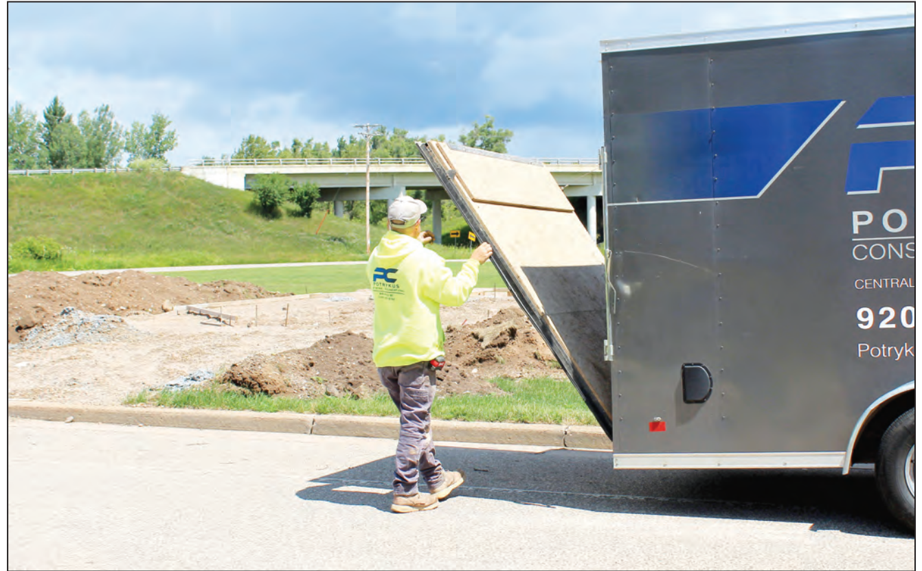
An employee of Potrykus Construction begins the day's work on the Wittenberg American Legion Post 502's veterans wall project. The idea has been bandied about for years, and, if all goes well, it will be finished in the coming months at a $70,000 cost.
