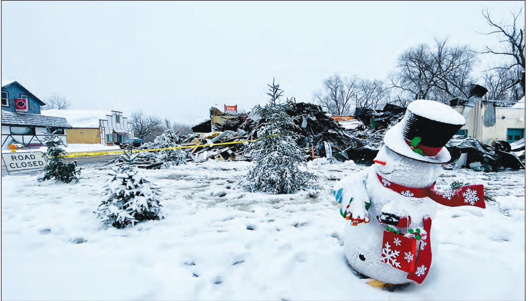
A fire on Feb. 23 in downtown Gresham obliterated this building, as wintry weather and other issues prevented the Gresham Fire Department from putting it out quickly. It's the second major fire Gresham dealt with in February.
