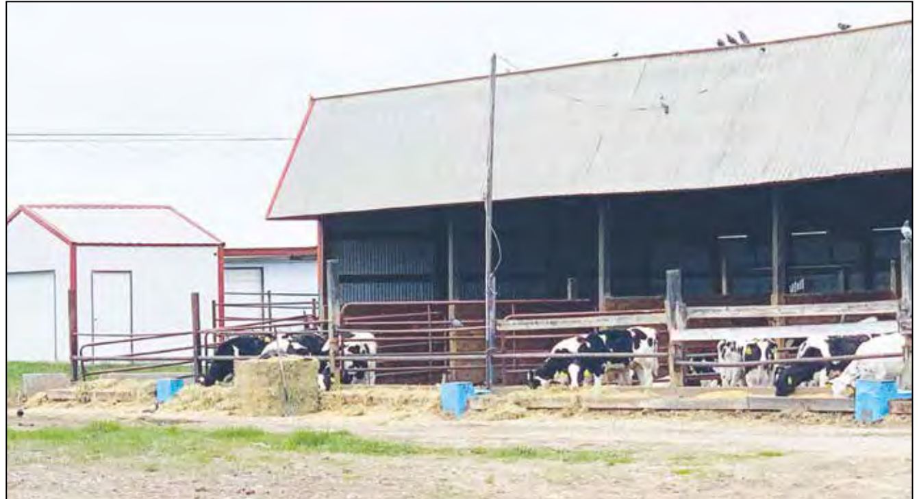
The expansion of Strassburg Farm would include upgrading from 1,650 animal units to 2,530 animal units. Animal units are measurement of how an animal affects a farm in terms of food and waste.
