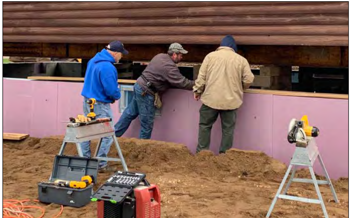
Dave Humblet, from left, Jeff Johanning and Rich Olson help level the foundation on April 24 for the Birnamwood American Legion post building. Humblet and Olson are among the volunteers who spent their Saturday morning prepping the structure.
