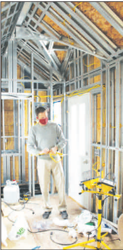
Caleb McPhail, building trades teacher at Wittenberg-Birnamwood High School, does a bit of tidying up inside the tiny house that is nearing completion outside of the school's shops. The project will soon join similar buildings from six Missouri high schools in Leadville, Colorado. The seven structures will be part of a rental complex in the mountain town.
