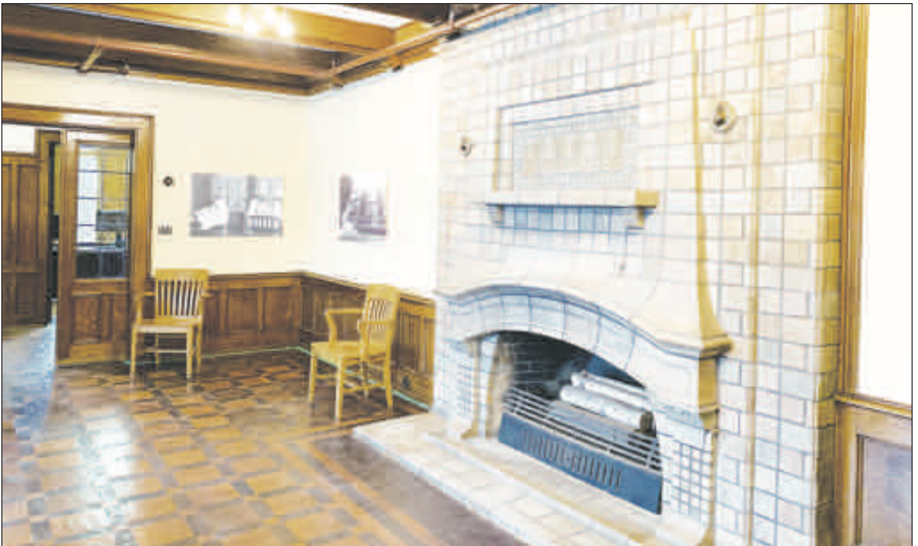
The waiting room at ThedaCare Family Medicine - Tigerton awaits patients. The village's clinic reopened Jan. 18. Patients will find the doors restored and paint on the windows removed, the original cork flooring revealed and the massive fireplace done in the Batch Elder style cleaned.
