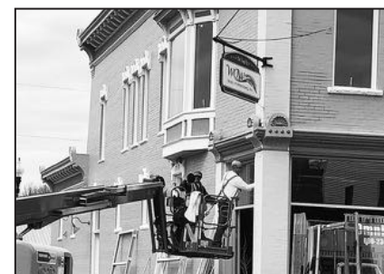
Good weather on April 6 and 7 helped make the installation of new window frames at the WOWSPACE in downtown Wittenberg an easier task for WOW workers Steve Vera and Dan Wisotzke.
