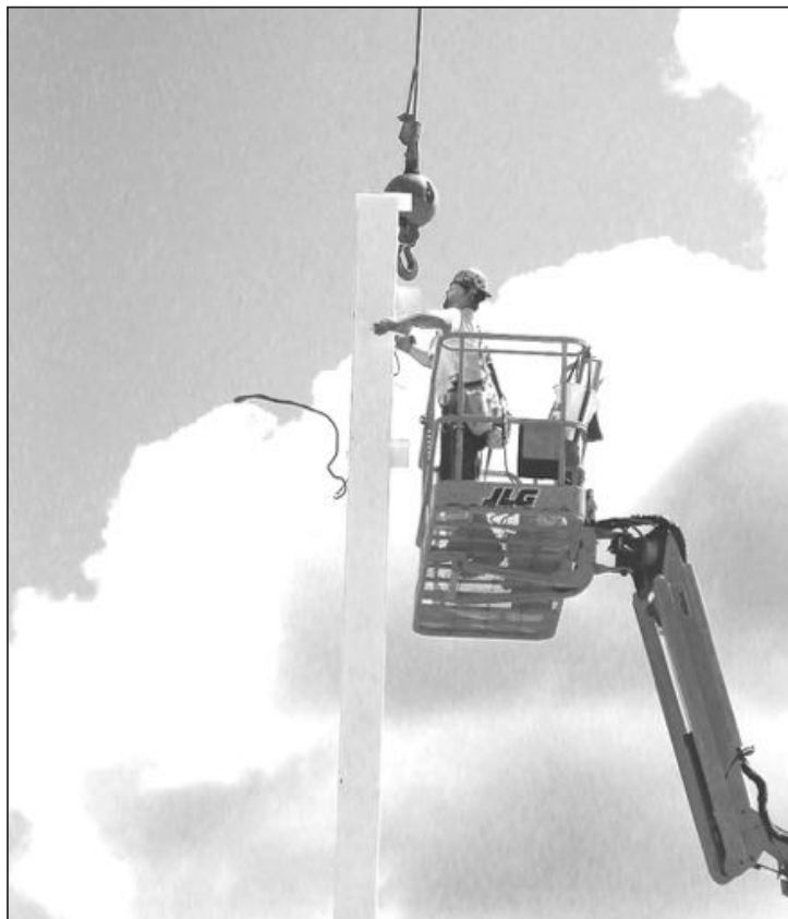
With the beam bolted in place, a SPE worker releases the belt. A white metal beam, signed by many of those watching its installation, is part of the Reinhart Food Service expansion project.
