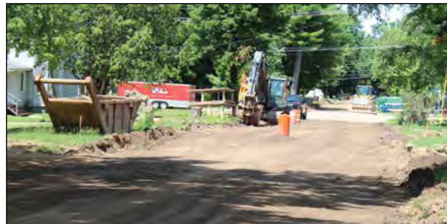
Weed Street is already torn up in anticipation of the work that will take place during the next eight to 12 weeks. The project will be a total reconstruction of the roadway — including pavement, base course, sidewalk, curb and gutter, as well as the utilities to include the water main, sanitary sewer and storm sewer.
