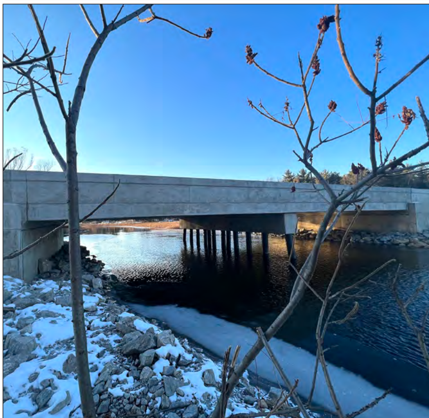
A newly constructed bridge sits on County Road HHH in Shawano. The bridge was rebuilt due to it meeting its life expectancy. The bridge features an upgrade the structure, including raising the bridge and adding room for foot and boating traffic.
