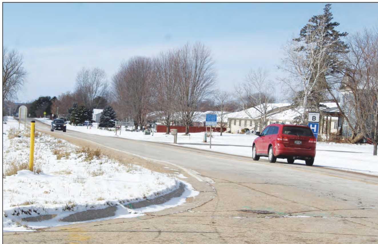
County Road B from Waukechon Street to Main Street will be one of the road reconstruction projects that the city of Shawano will be working on during 2023.
