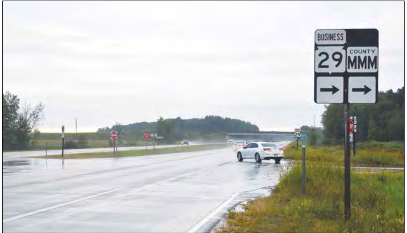
The state Department of Transportation is proposing a J-turn among four alternative to upgrading the intersection of state Highway 29 and County Road MMM west of Shawano, but the Richmond Town Board wants the state to consider building on- and off-ramps to the Maple Avenue overpass, which can be seen in the distance in this photo.
