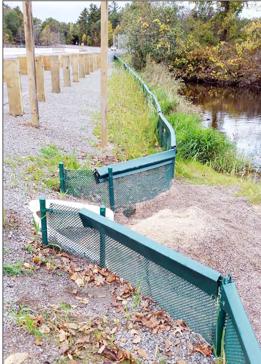
A crossing structure in Portage was built to allow wildlife access without requiring them to cross busy roads.
