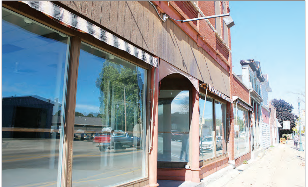
The 200 block of North Main Street in Shawano has been largely empty of businesses for about 18 years. Officials for the city, which recently purchased the buildings, believe three out of four of them can be renovated.
