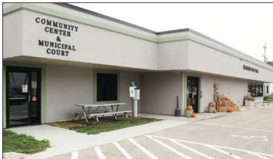
Shawano City Hall is closed to the public, along with most key city facilities.
