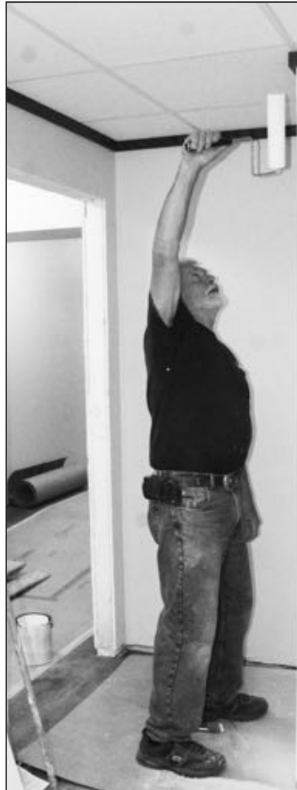
Larry Laude applies some of the finishing touches on the paint for one of the rooms nearing completion at the SAM25 homeless shelter on East Richmond Street in Shawano. His construction company is among those making the renovations. Also involved are Knope Heating & Cooling, Mode & Sons Plumbing and Radtke-Reuter Electric.
