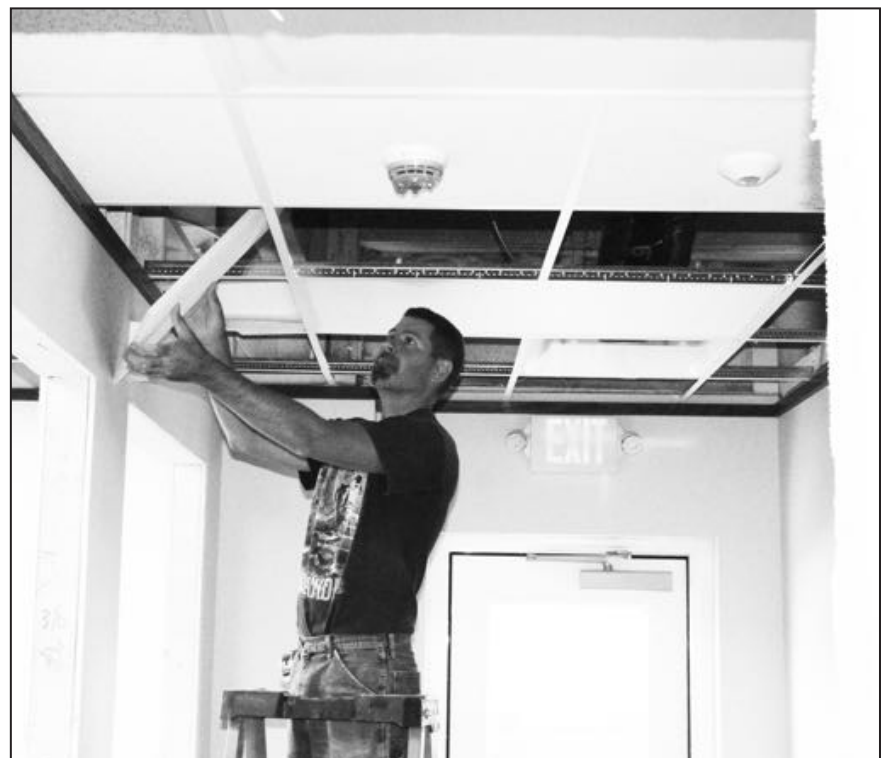
Joe Schmude fits a ceiling tile near the entrance of the soon-to-be-renovated SAM25 homeless shelter on East Richmond Street in Shawano. He works for Larry Laude Builders, one of the contractors working on the building.
