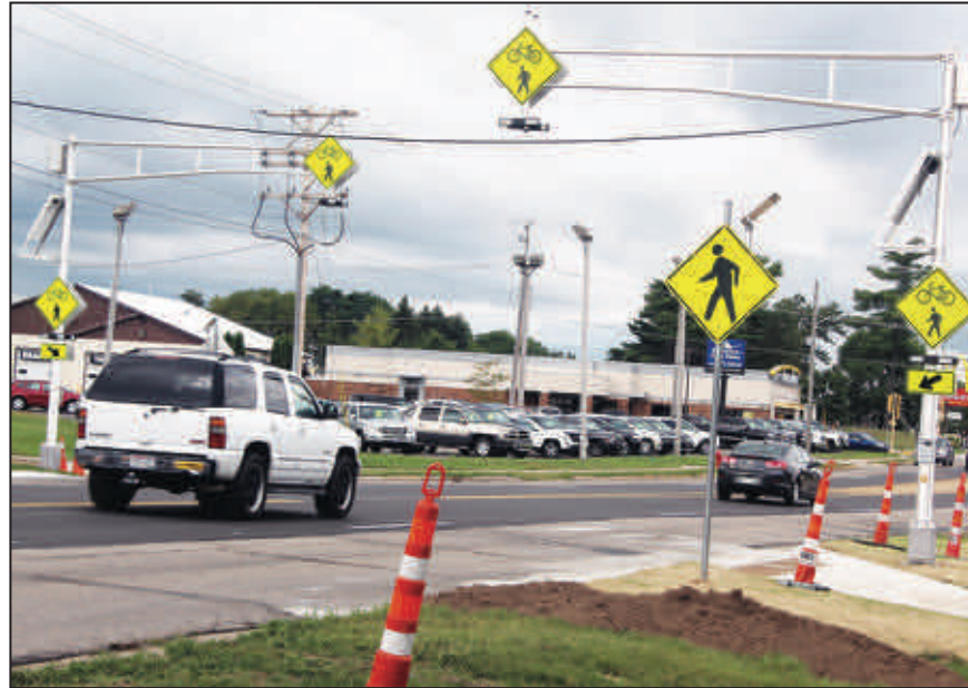
Vehicles travel Monday underneath the new mast arms signalling the Mountain Bay Trail crossing on Green Bay Street. When hikers and walkers plan to cross the street, they will press a button that activates the warning lights so motorists know to stop.
