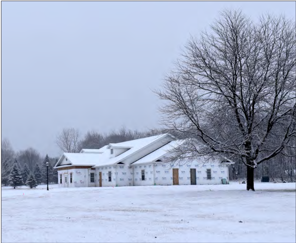
Renovation of the former Kaempfer and Associates building continues at 650 E. Jackson St. in Oconto Falls, where the goal is to open an Encompass Child Care Center serving up to 140 children by mid-June.
